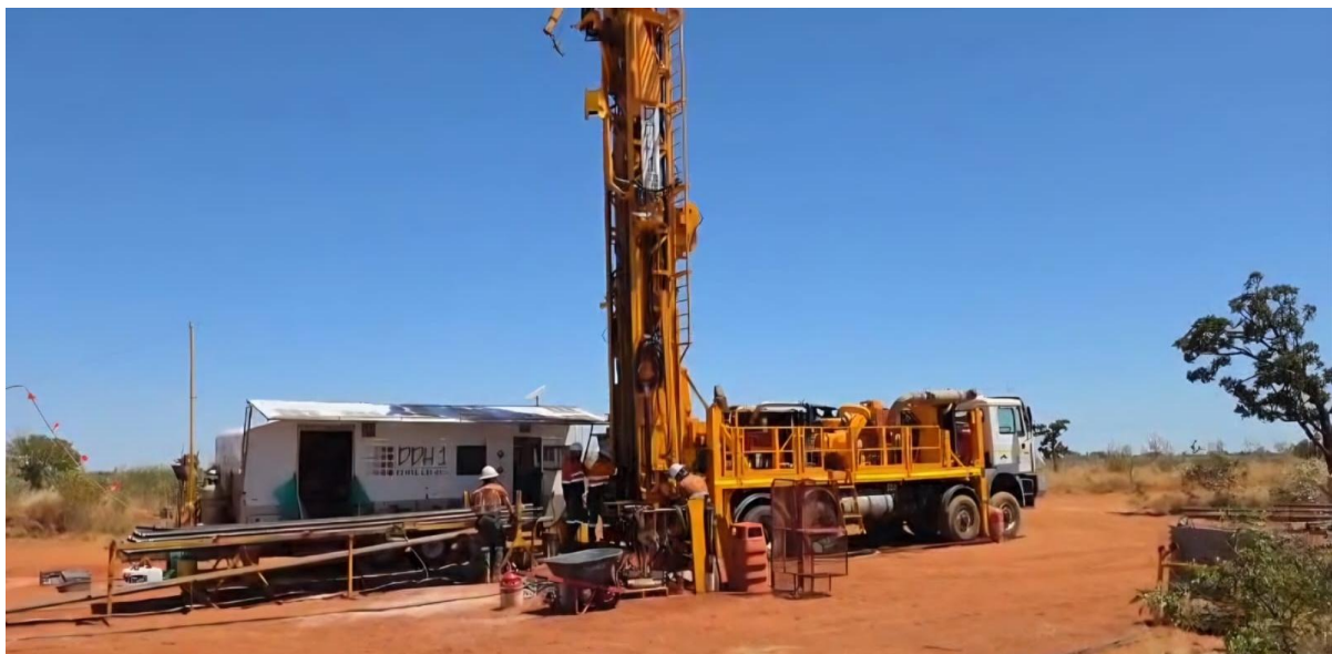
[Figure 1] Pulkarrimarra drilling in progress
