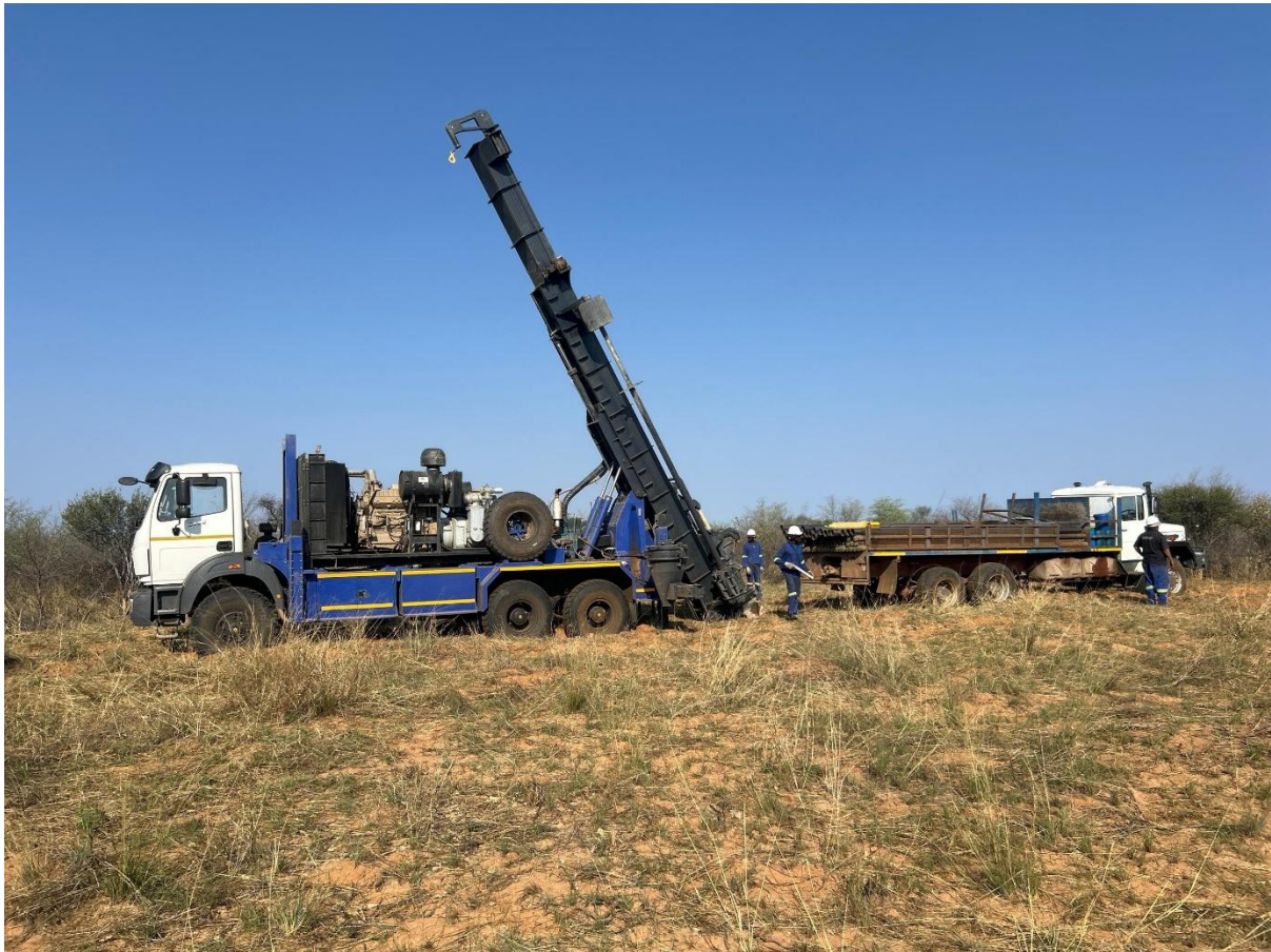
Figure 1: RC drilling commences at the Powerline Project
