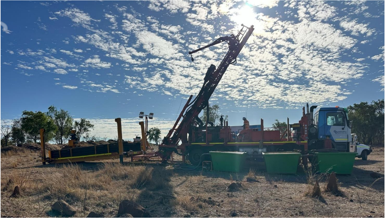
Figure 1: Drilling contractors Geo Drill Australia on site at the Mt Turner Gold Project in Queensland, Australia
