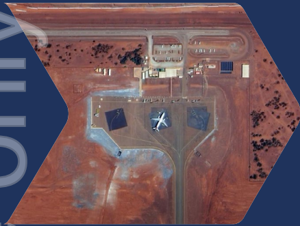
Electrical and communications works for Ginbata Airport in Newman, WA.
