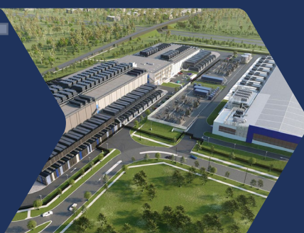
Electrical and communications works for AirTrunk hyperscale data centre, Melbourne, VIC.
