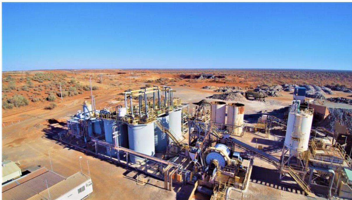
Figure 2 - Burnakura gold processing plant
