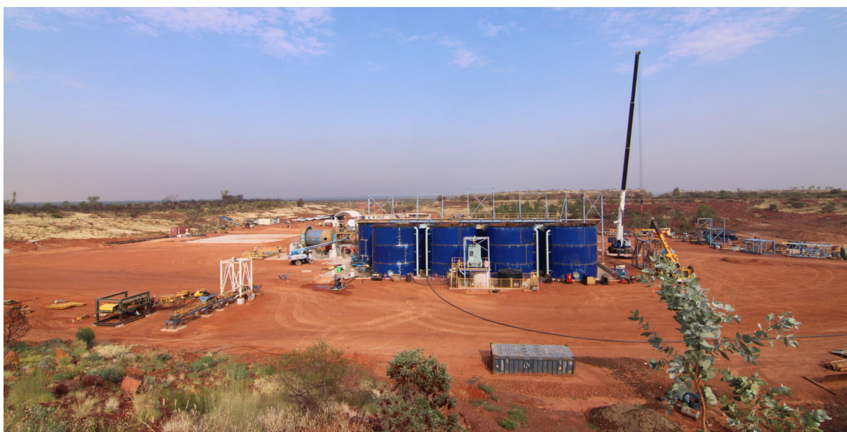
Construction of Nobles CIL Gold Processing Facility 2024
