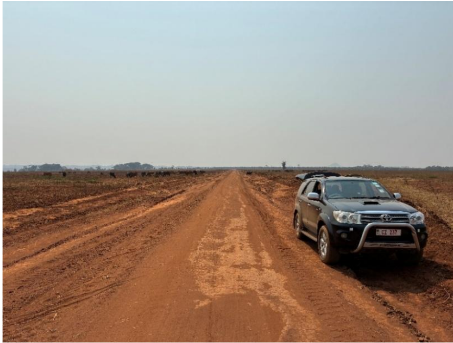
Figure 3. Graded road access within the project area
