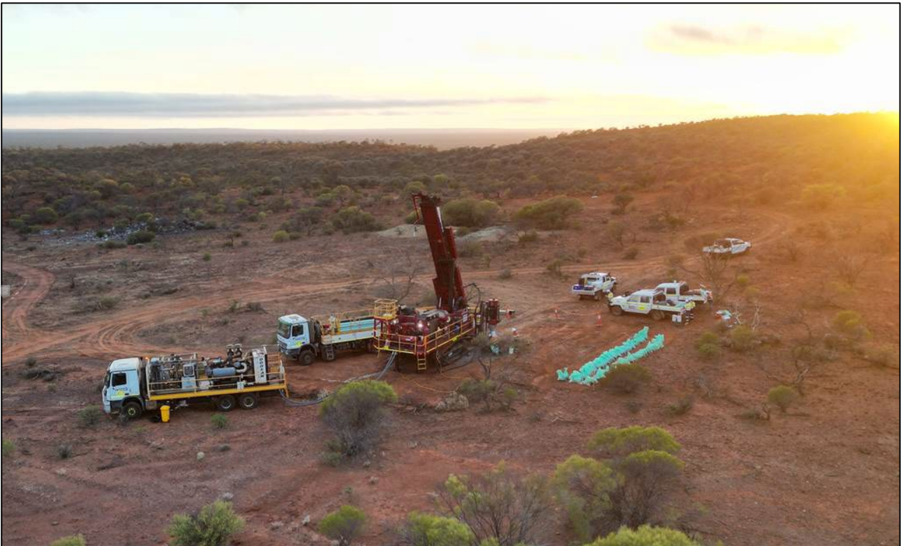
Figure 3: Drill rig at Wadgingarra, Yalgoo Project
