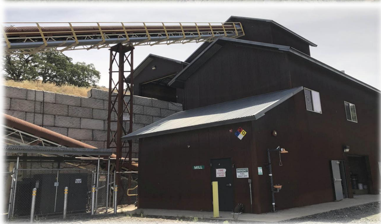
Photographs: Infrastructure at the Lincoln Gold Project.
