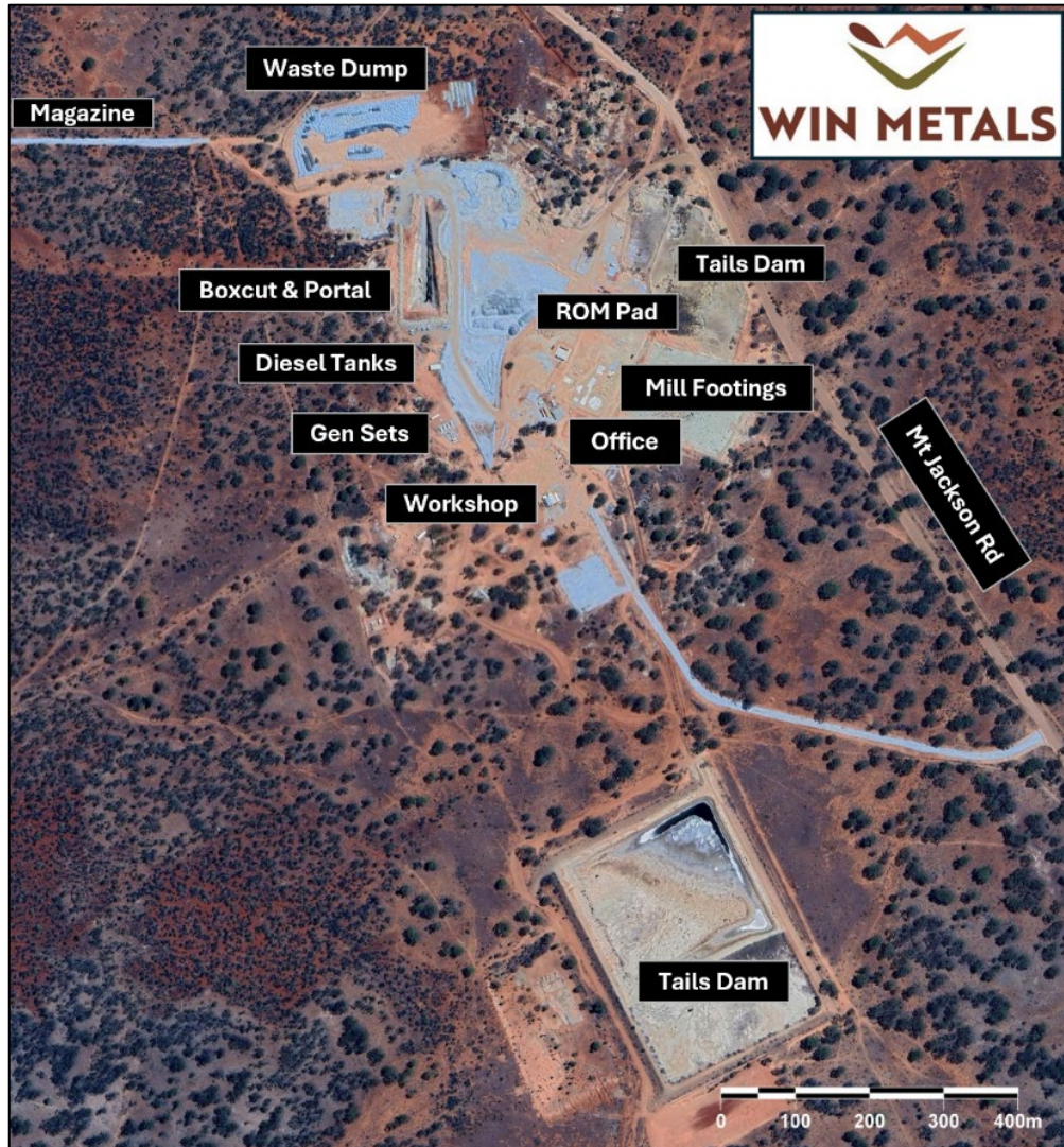
Figure 2: Radio Mine Site Infrastructure
