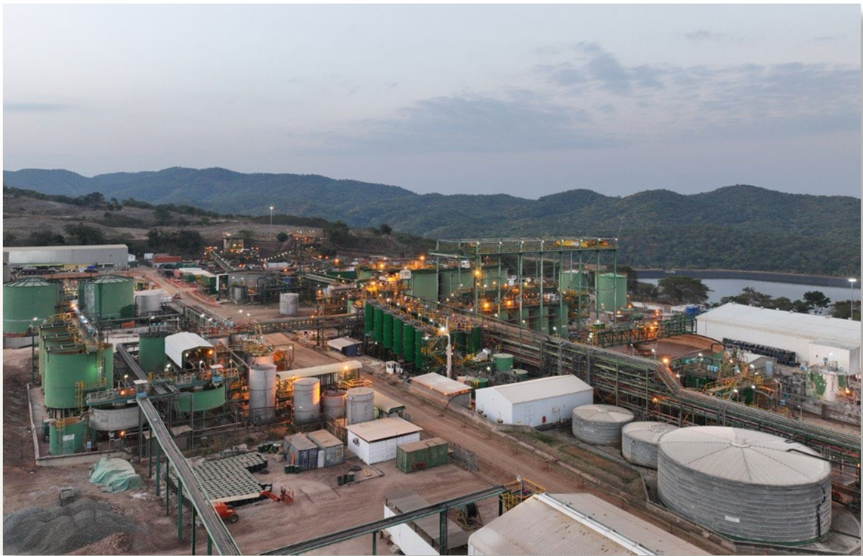
Figure 2: Kayelekera process plant (back end) during commissioning
