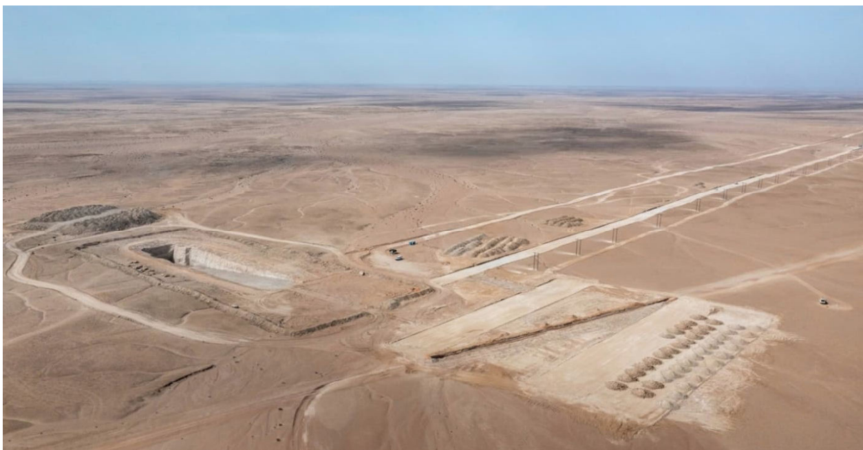
Figure 2: Significant progress continues on bulk earthworks at Etango, a key enabler of future construction and development activities. The primary crusher has been fully excavated and its dimensions confirmed, while work advances on the permanent road and conveyor belt line to the secondary and tertiary crushing areas.
