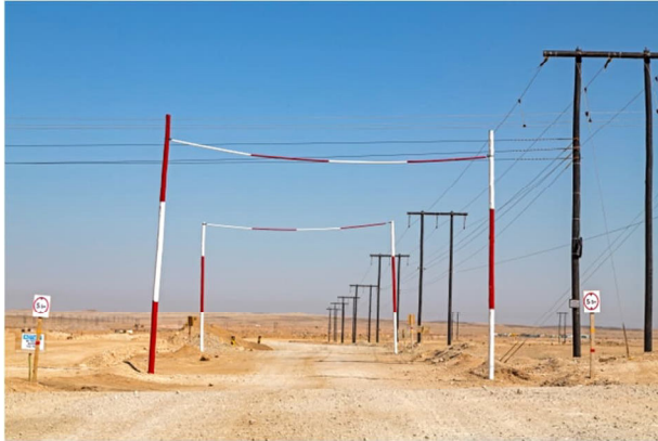
Figure 4: Power grids on site are now live with safety precautions to prevent vehicles crossing under installed lines
