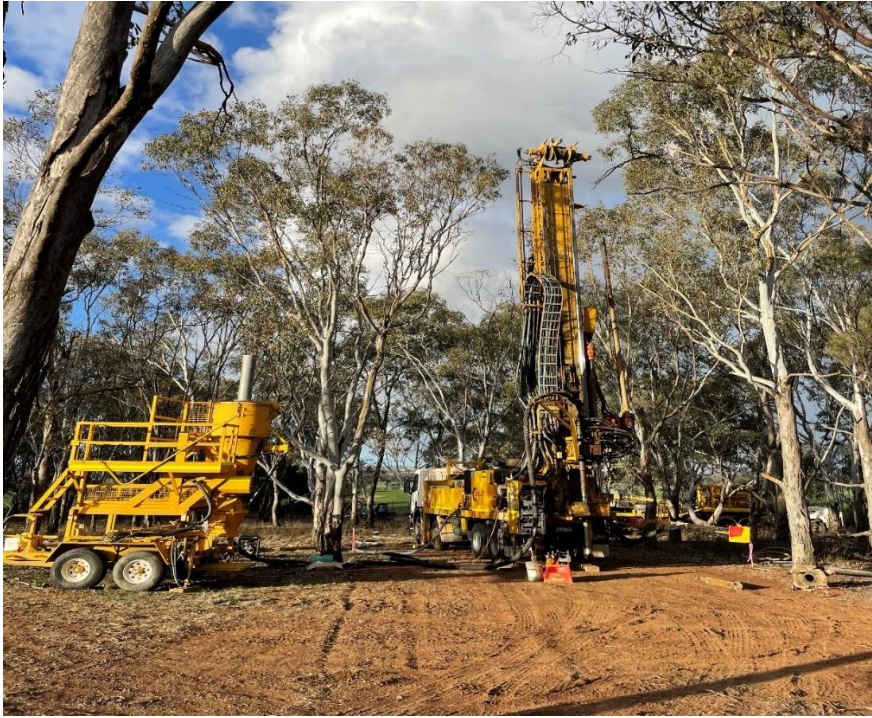
Figure 4: Drill Rig mobilised at Gidginbung gold deposit (July 2025)
