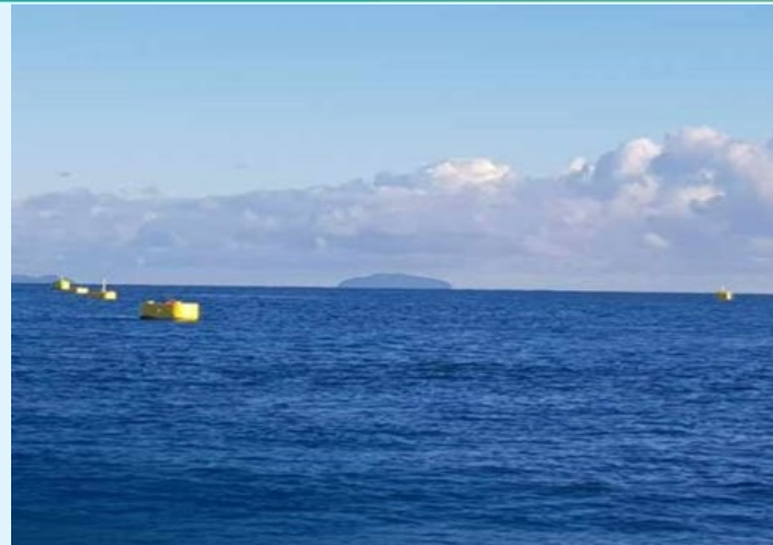
Blue Endeavour mooring grid work underway
