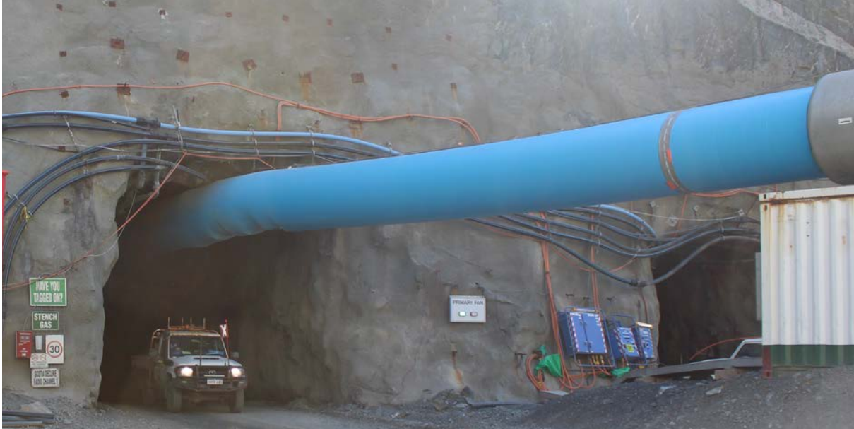
Picture – Scotia Underground Mine, South Portal.
