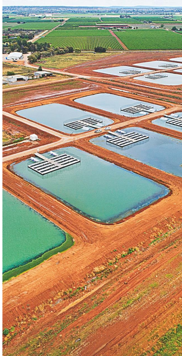
Overhead view of our Bilbul Site
