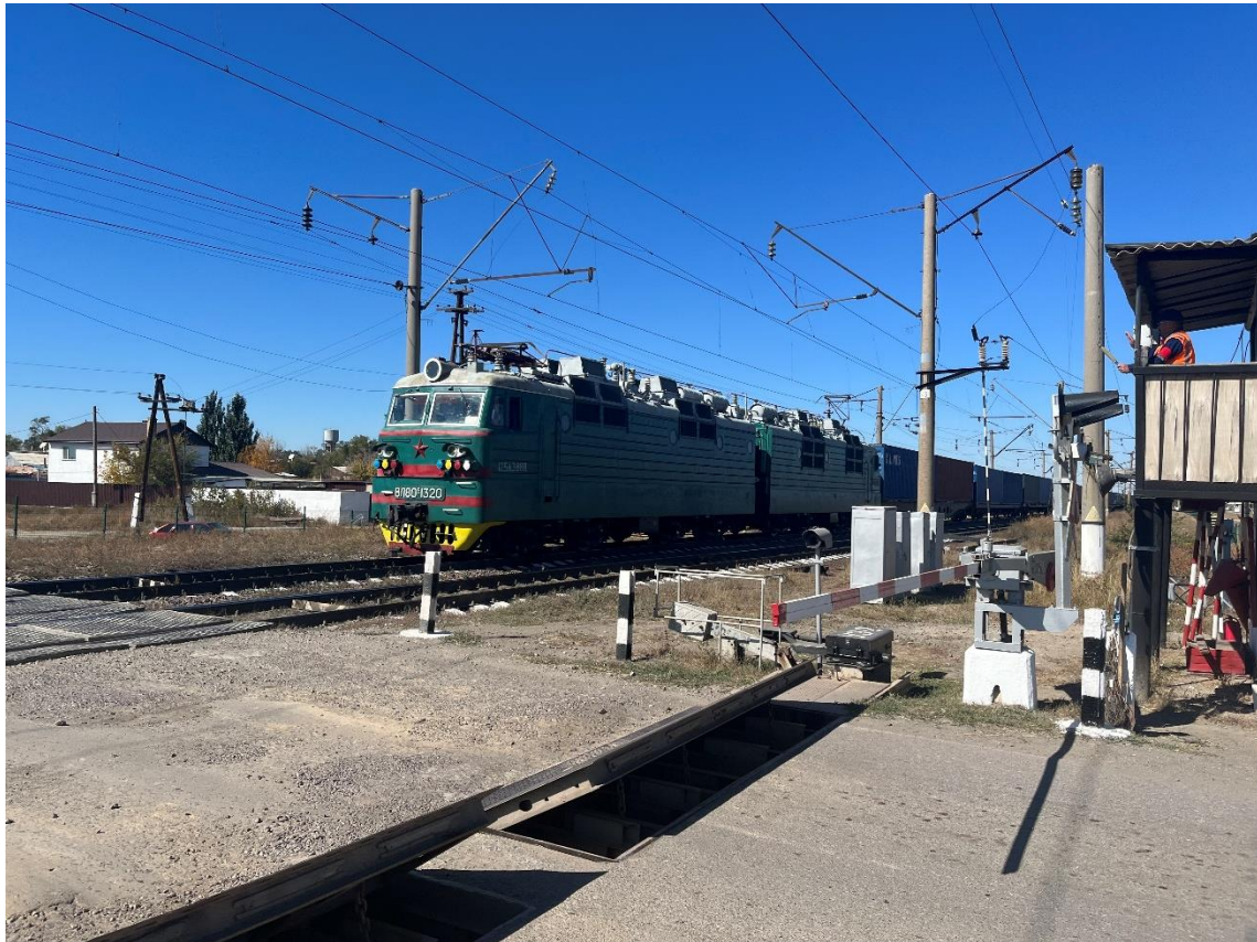
Figure 9 - Electrified heavy haul railway crossing in Agydyr, Kazakhstan
