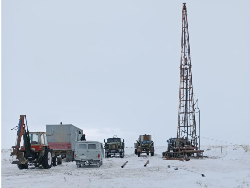
Figure 5 – Water bore drilling underway in the Sherubainura River Aquifer
