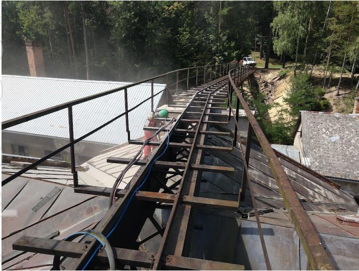
Image 3 (left): cleaning and painting the rail link bridge over the engine room; Image 4 (right): near complete roof repairs and installation on the engine room at the Sturec project;
