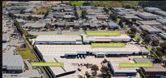
WETHERILL PARK NSW
