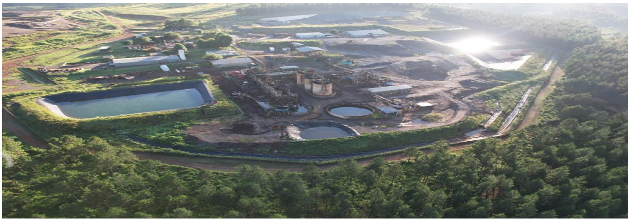
Figure 6: District view of TGME Processing Plant, Workshops and Tailings Dam prior to de-commissioning
