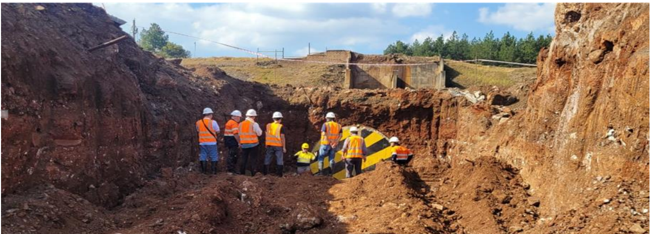
Figure 4: General Team Discussion Regarding Future Plant Equipment Installations
