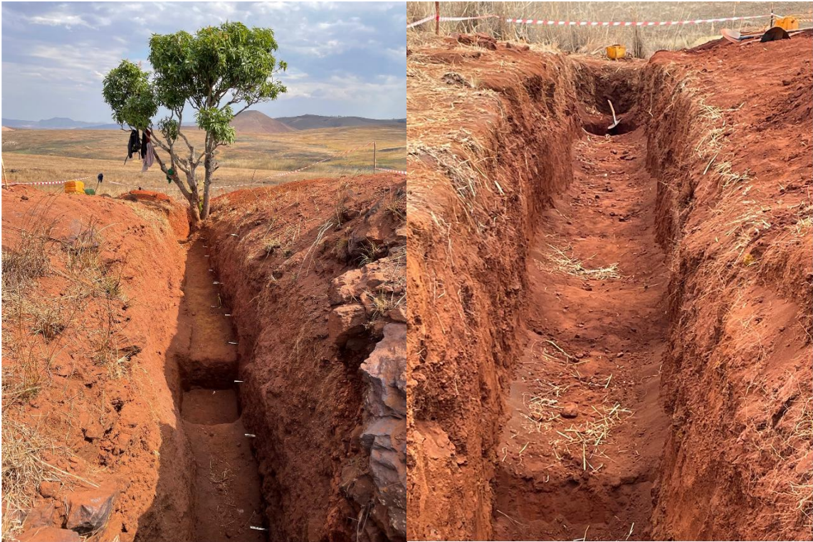
Figure 3 Bekisopa Trenching – 2025 program in progress
