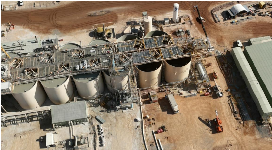
Figure 2: KoTH process plant upgrade with 4 new CIL tanks at full height
