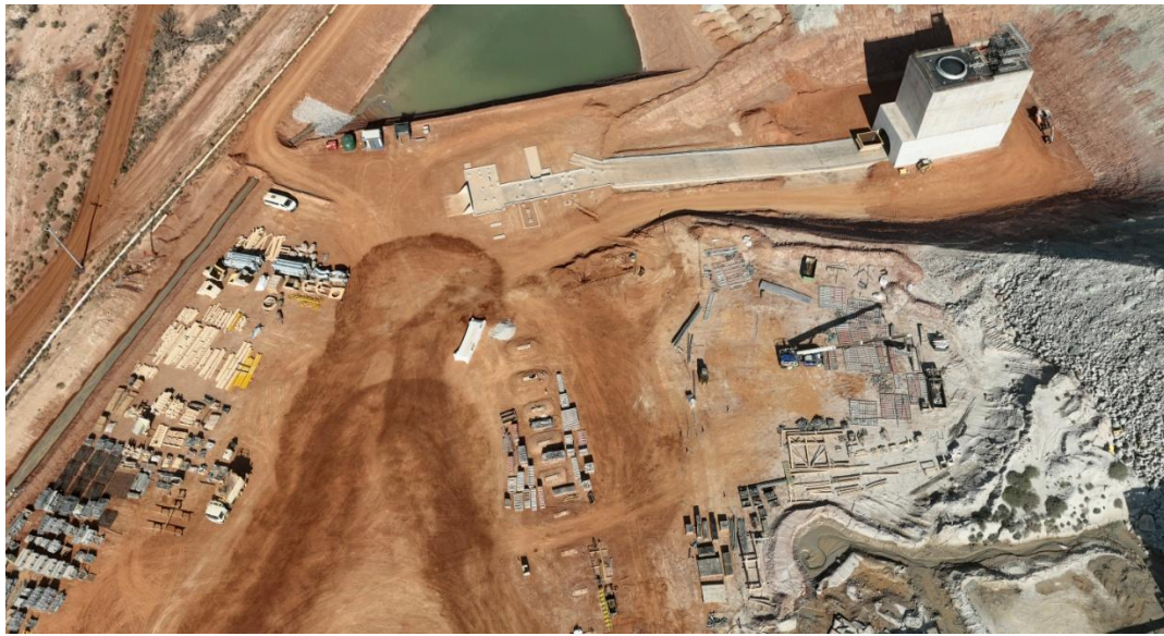
Figure 1 KoTH new primary crusher vault installation
