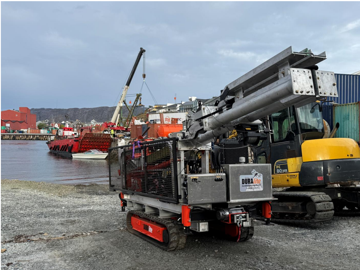
Figure 1: Loading of Diamond Drilling Rig and Support Equipment onto Transport Barge in Qaqortoq Harbour
