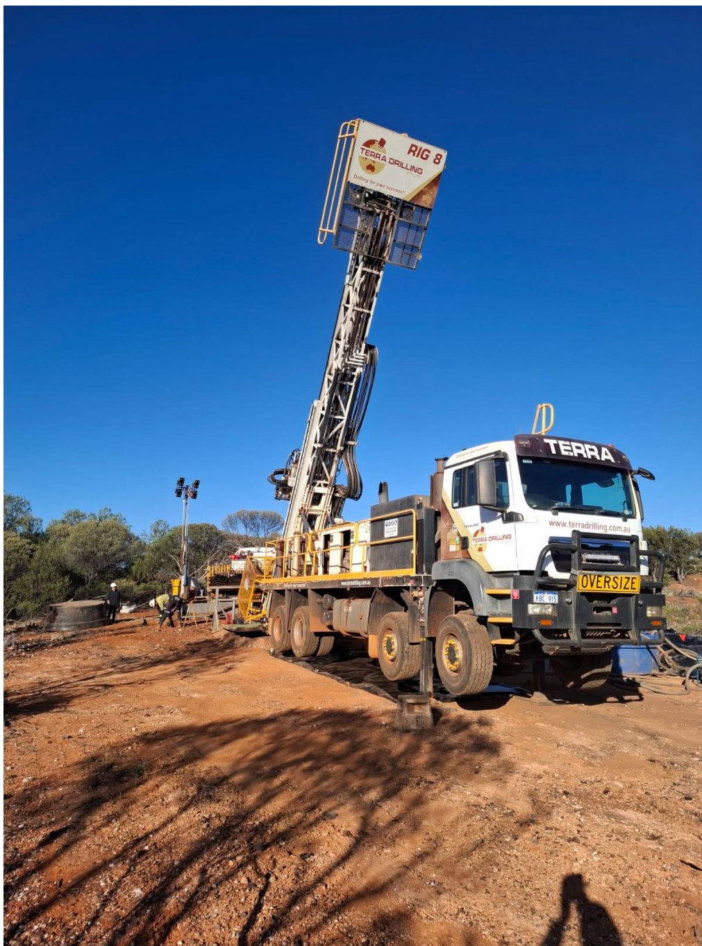
Above: Diamond drill rig on site.
