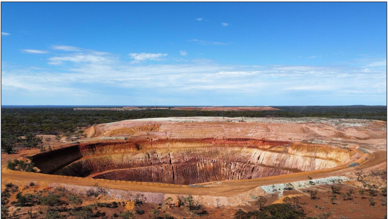
Figure 1. Eureka Gold Project – Current Eureka open pit, aerial view looking east. Note the excellent wall condition
