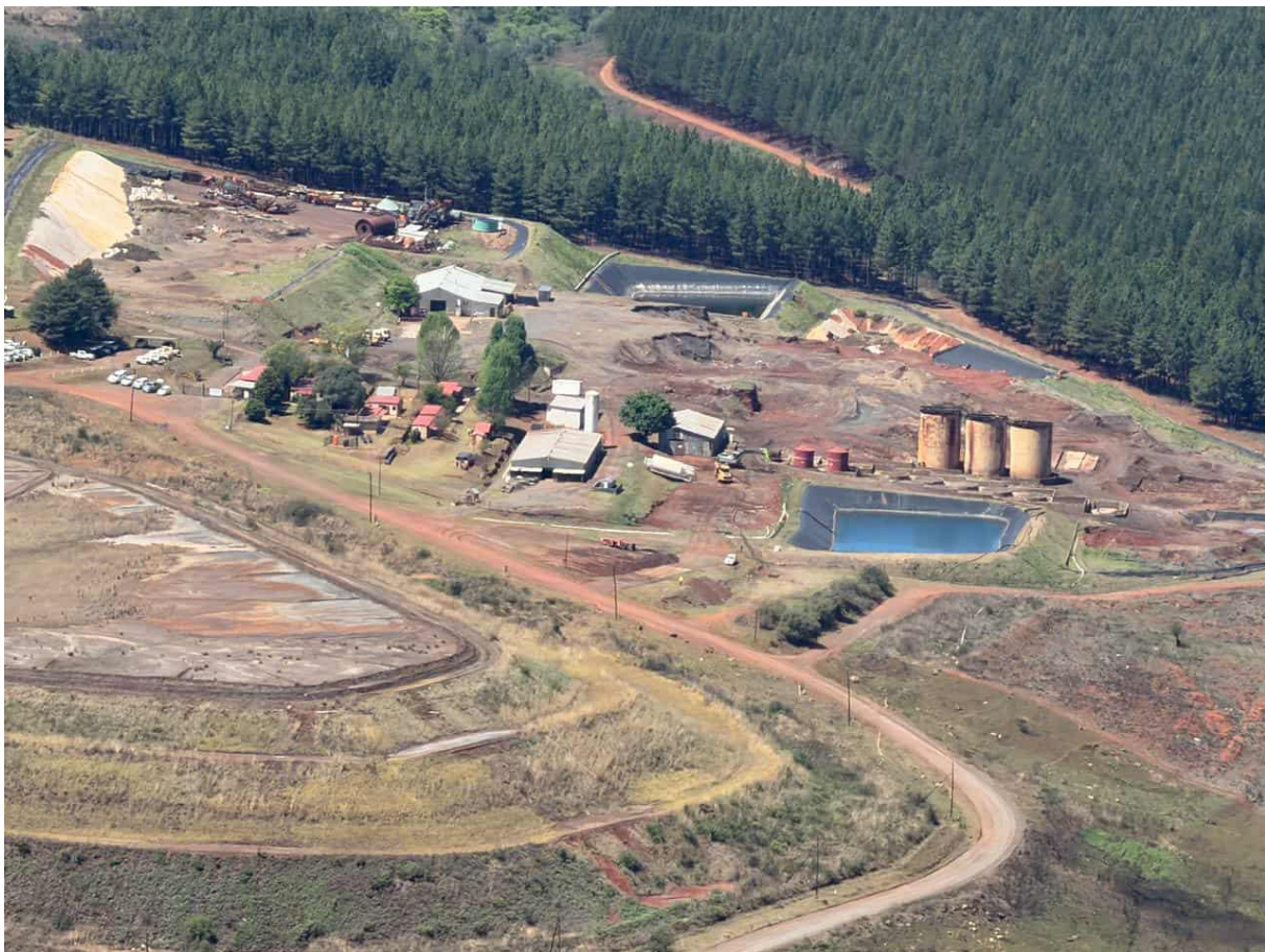
Figure 1: Aerial photo of the exiting Plant post decommissioning of old facilities.
