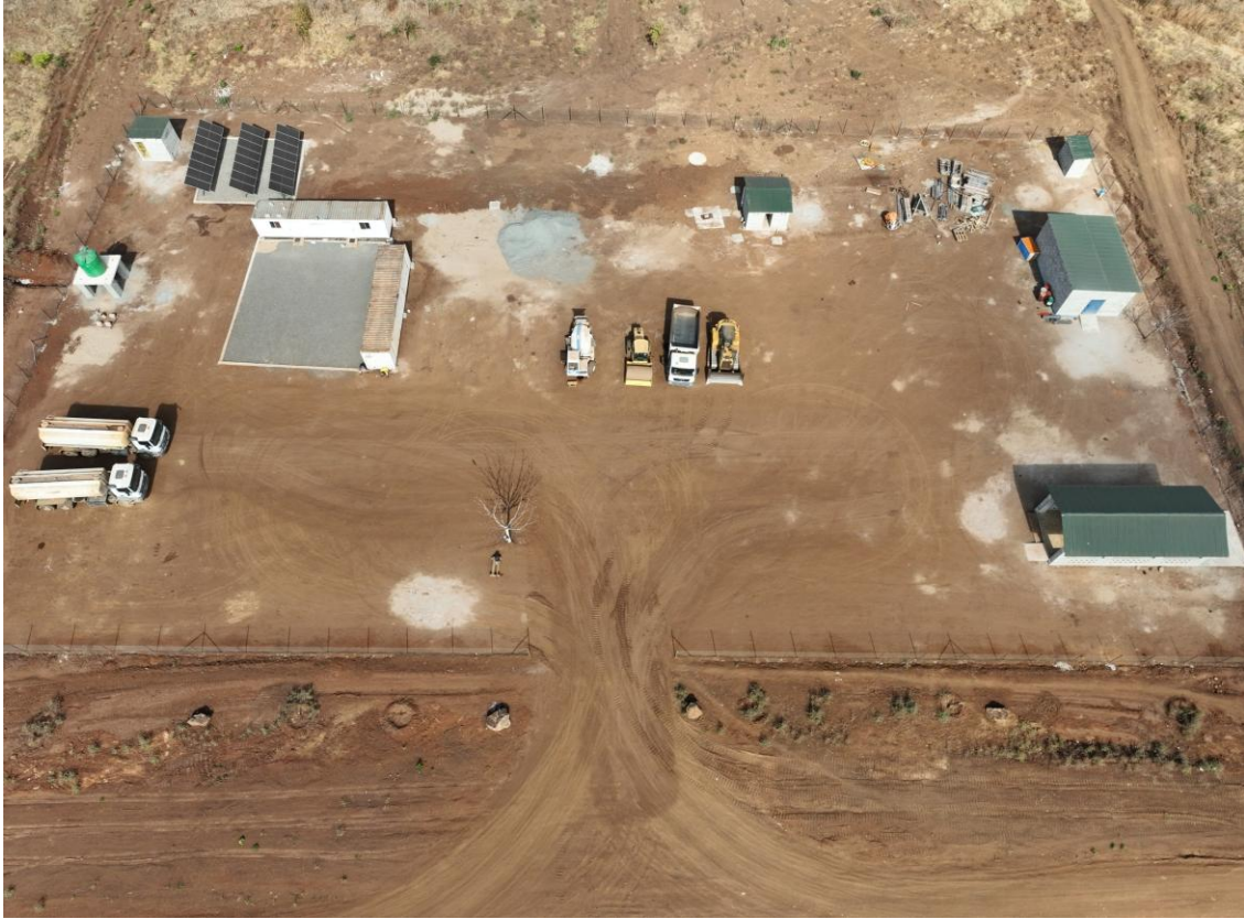
Picture 3. Contractors' laydown area at Kangankunde.
