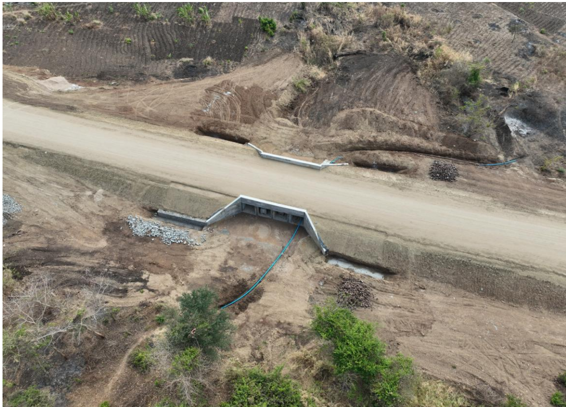
Picture 1. Completed culvert on site at Kangankunde.
