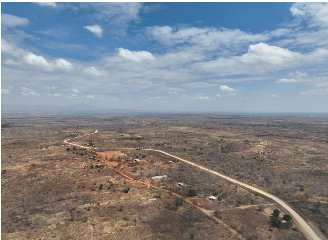
Picture 4. Main 5km access road at Kangankunde.
