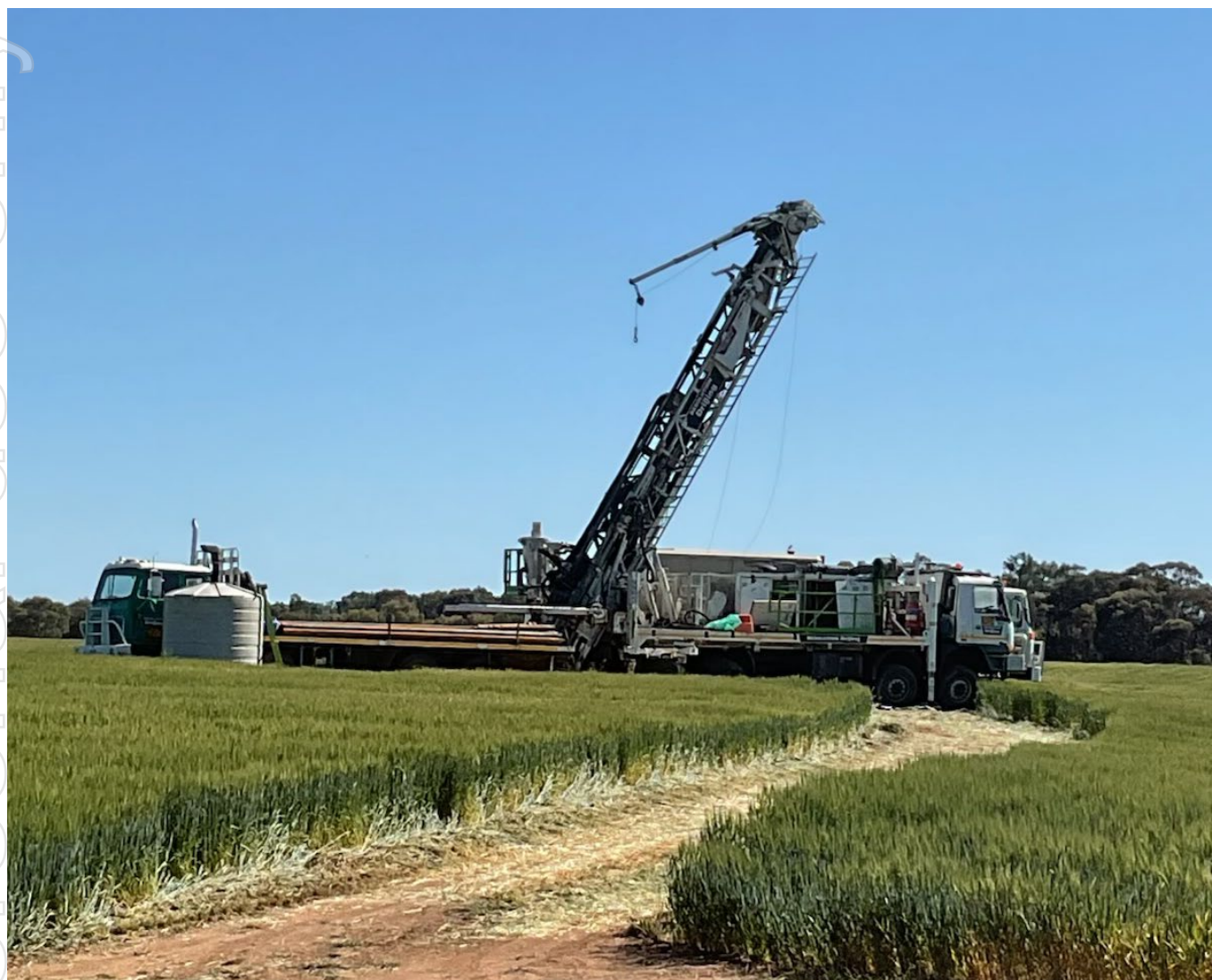
Figure 5: UDR1200 setting up to commence drilling at the Dam (October 2025).
