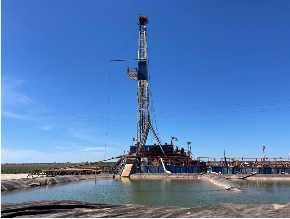
Photo 2. JVU-5 drill rig and lined pit.
