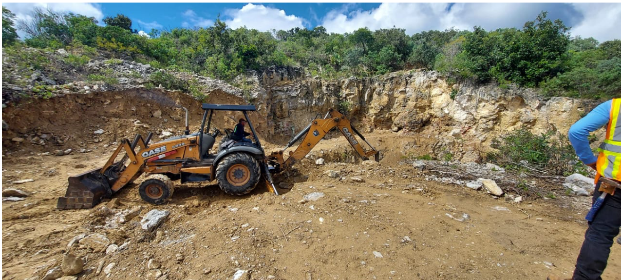
Clean up pits for fresh rock exposure
