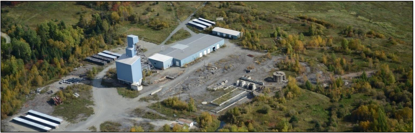
Figure 1 – Surface infrastructure at the Rouyn Gold Project in Quebec
