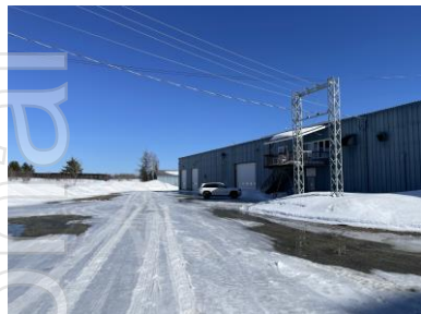
Site connection to hydro-power and major infrastructure
