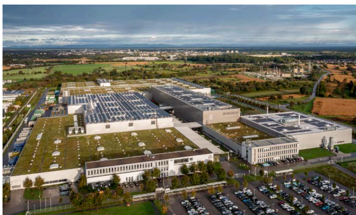
Figure 4 – Recycling Plant Building (far right) at Mercedes-Benz, Kuppenheim
