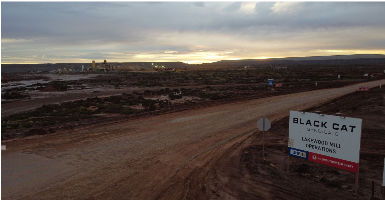
Figure 1: Lakewood processing facility
