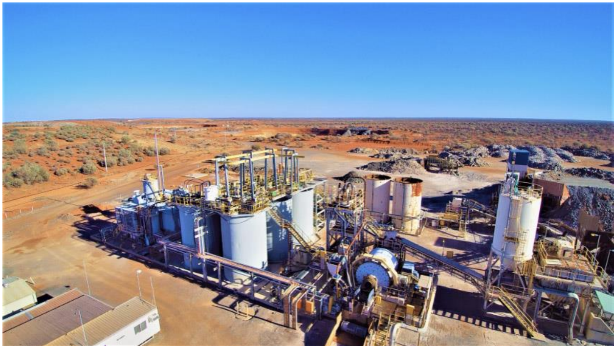
Figure 5 - Burnakura gold processing plant
