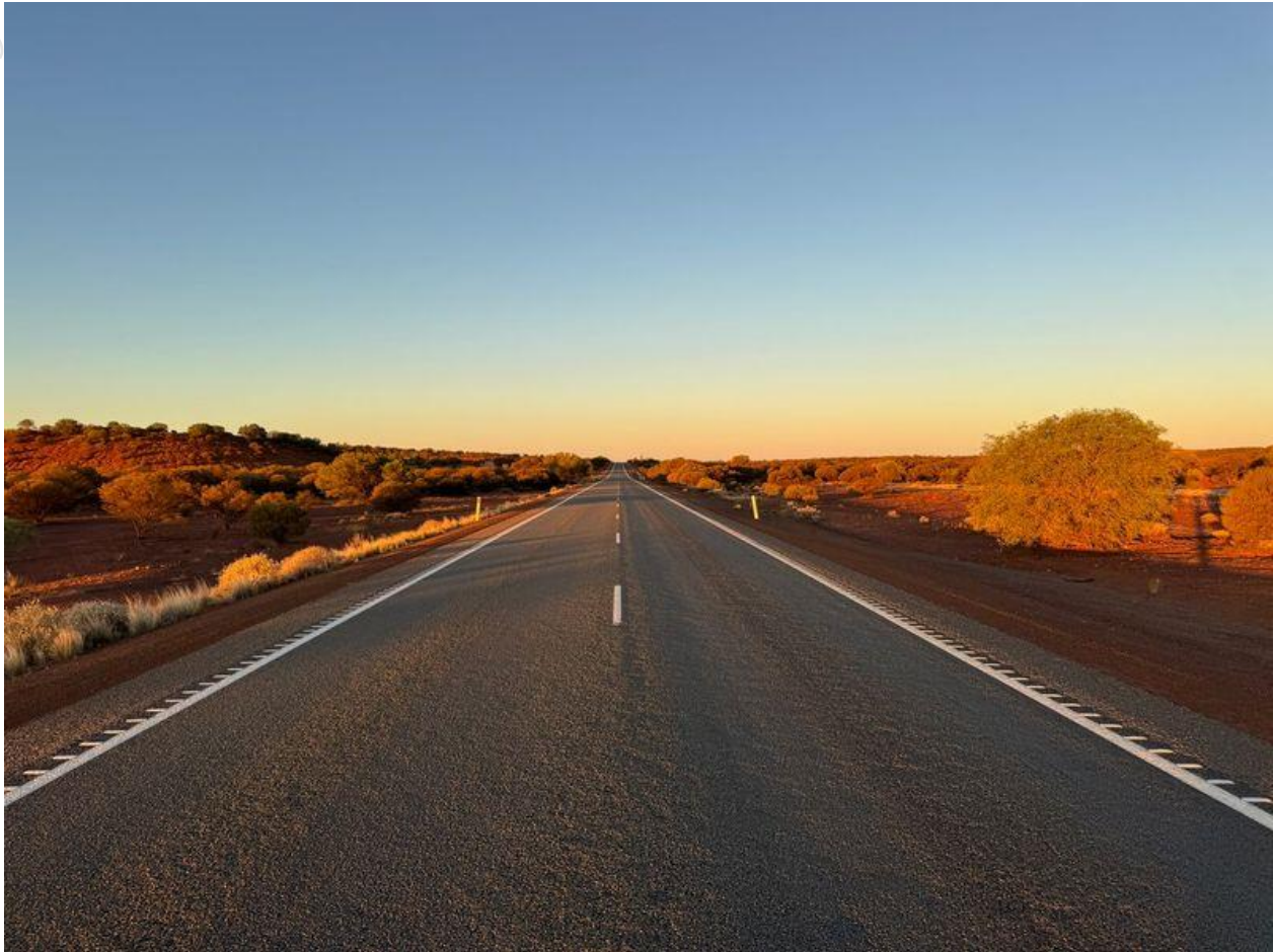
Figure 9 - Great Northern Highway looking North
