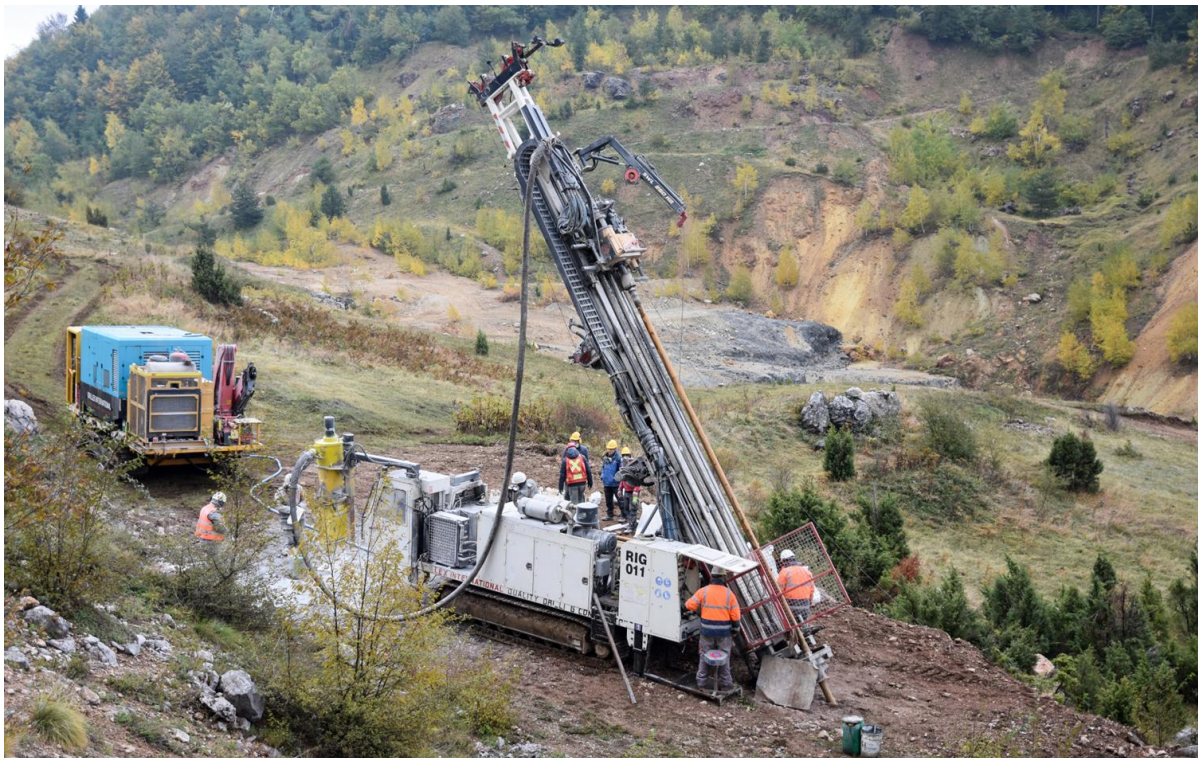
Figure 1 – Drilling in the historic Bobija open pit mine area (Oct. 2025).
