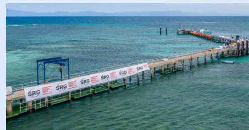
Green Island Jetty Remediation
