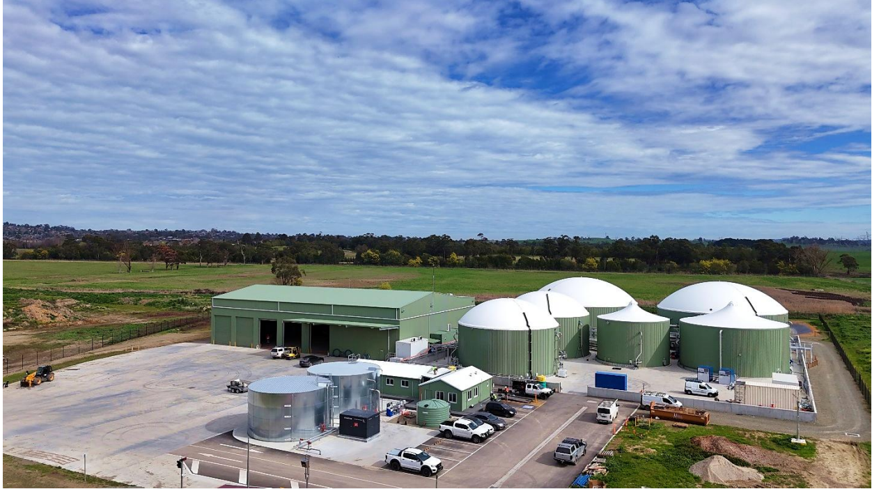
Yarra Valley Water Bioenergy plant in Lilydale
