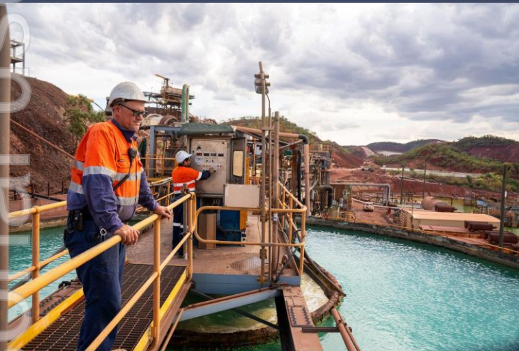
Processing plant & surface infrastructure
