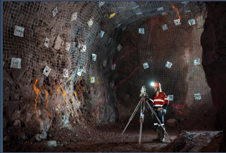
Established underground development
