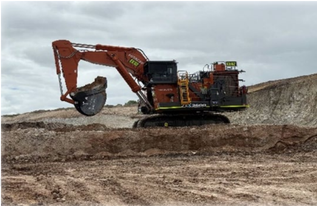
New EX3600-7 – First Bucket of Dirt
