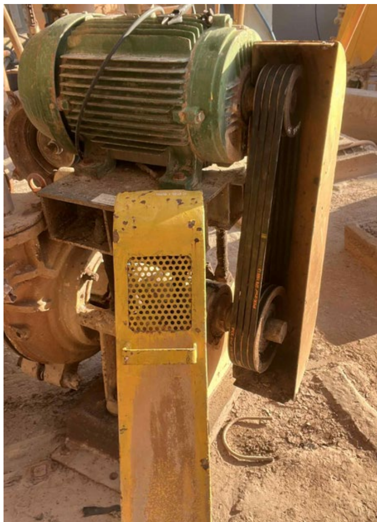
Figure 1: Mill pump belts replaced, adjusted ready to go.
