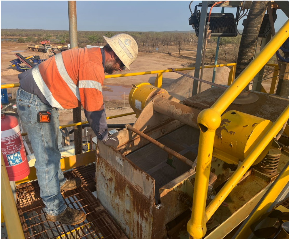
Figure 2: replacing the nelson scalping screen mat
