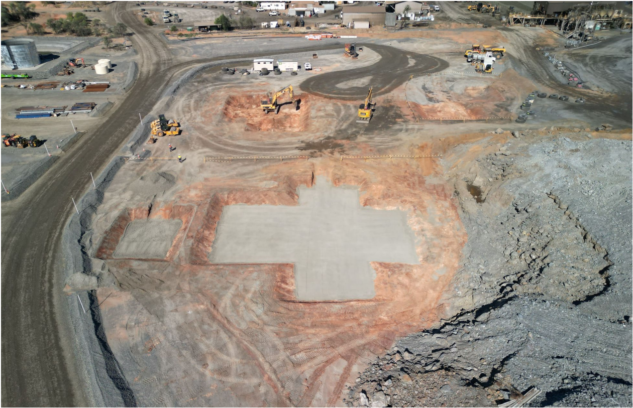
Photo: Foundation excavation for new crusher – process plant earthworks.
