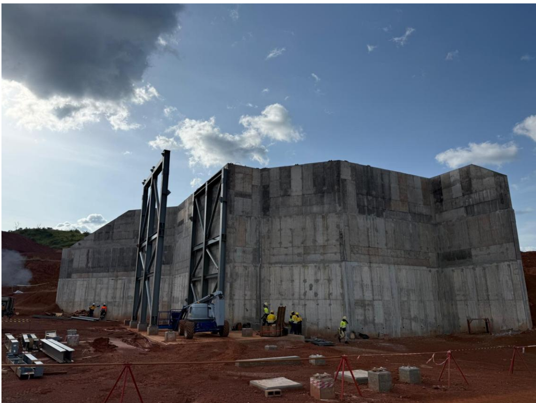
Figure 8: Oxide crushing steel erection progress (13 October 2025)
