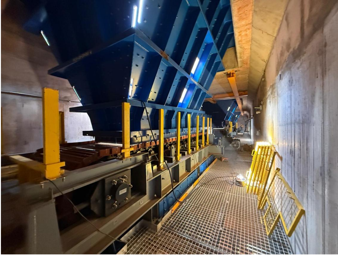
Figure 9: View of inside the reclaim chamber (13 October 2025)
