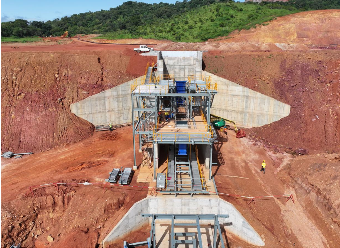
Figure 7: Primary crusher steel erection progress (11 October 2025)
