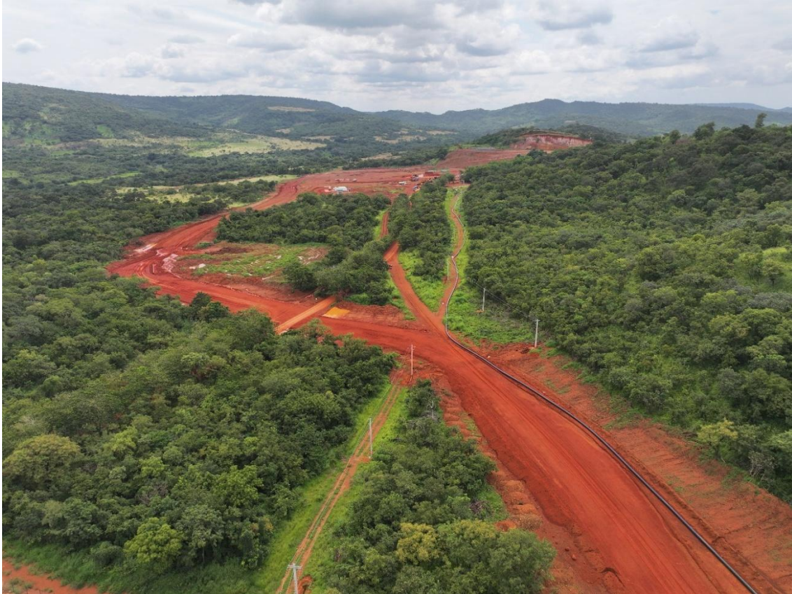
Figure 13: Overland piping installation (12 October 2025)
