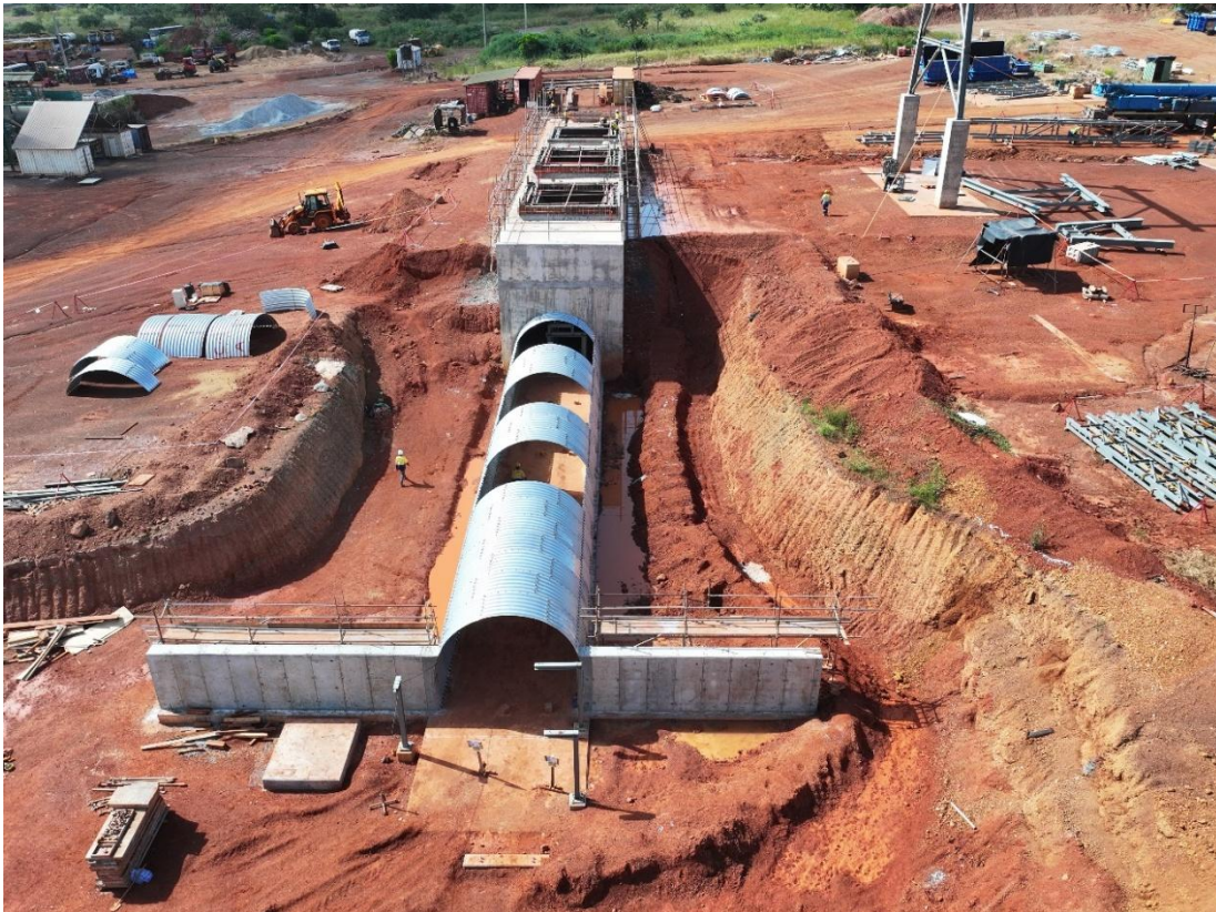
Figure 10: View of top of the reclaim chamber (11 October 2025)
