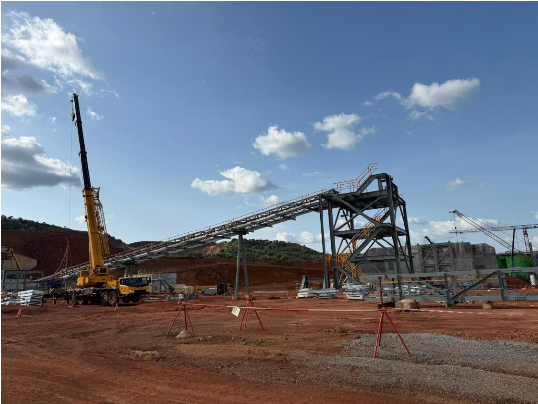
Figure 5: Stockpile feed conveyor truss modules erection (13 October 2025)
