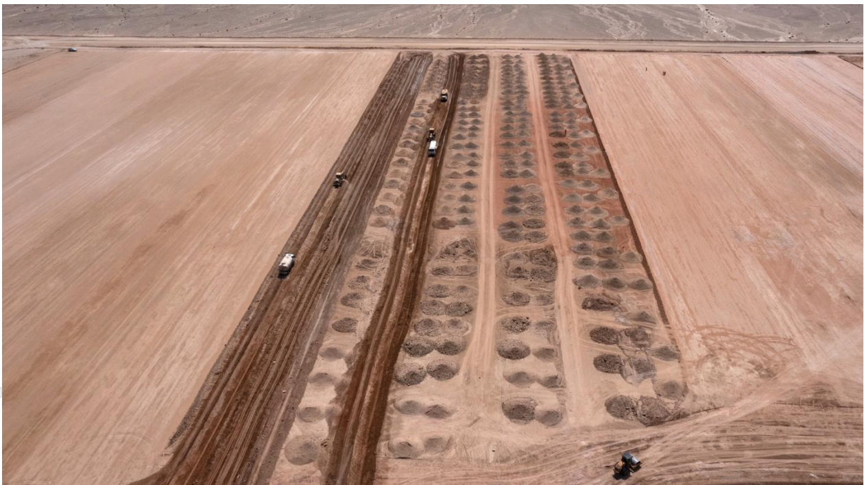
Figure 1: Heap leach earthworks continue to advance strongly.
