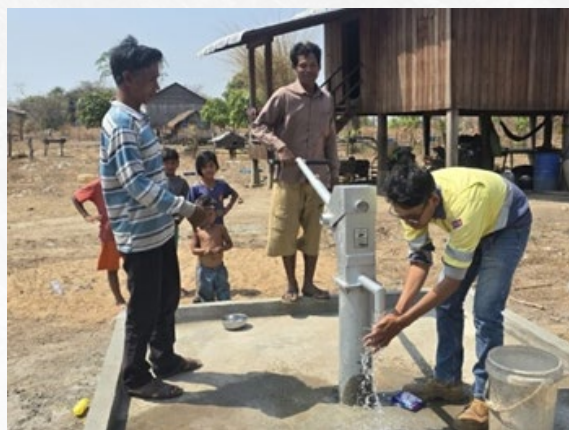
Figure 39 | Community water bore
