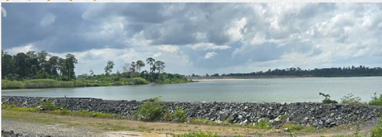
Figure 38 | Tailings Storage Facility at Okvau
