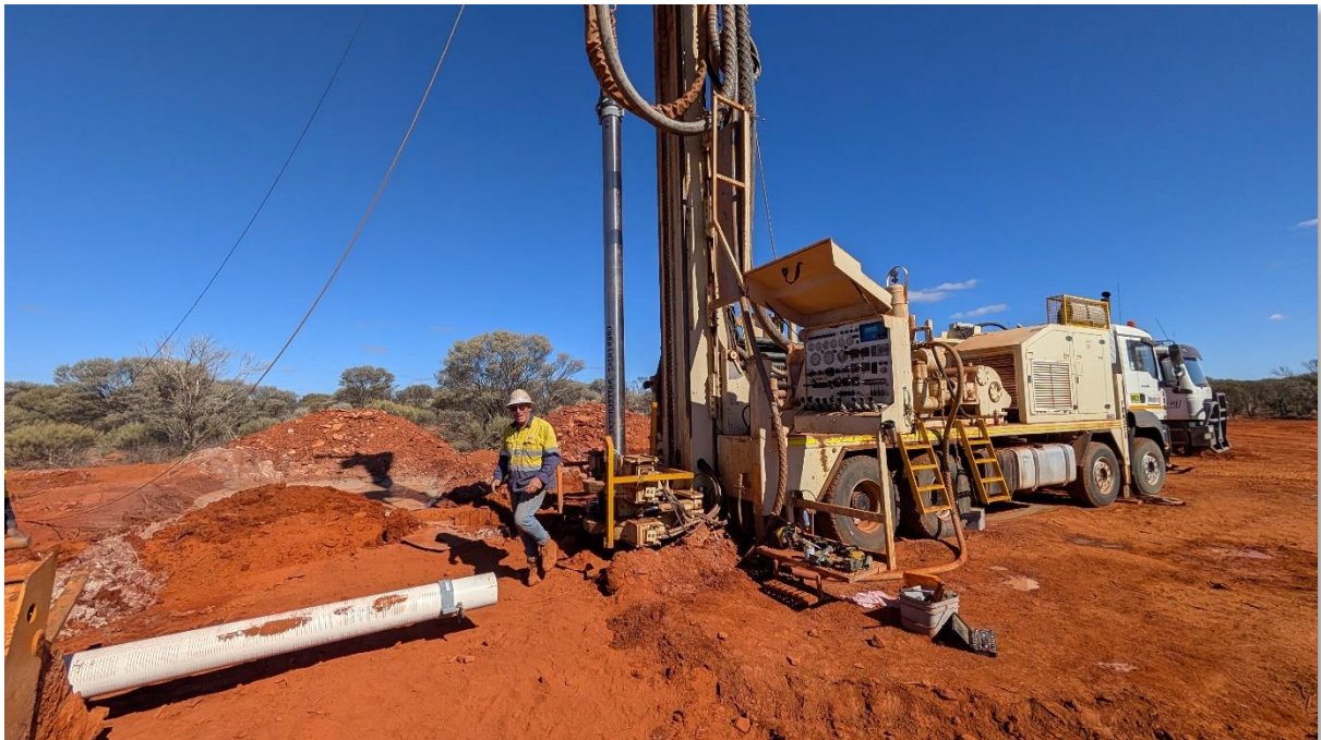
Figure 3 - Construction of production bore
