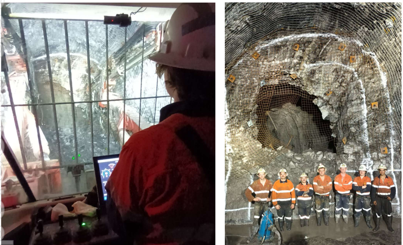
Figure 1 – Main Lode incline/decline breakthrough completed by the Byrncut development team.
