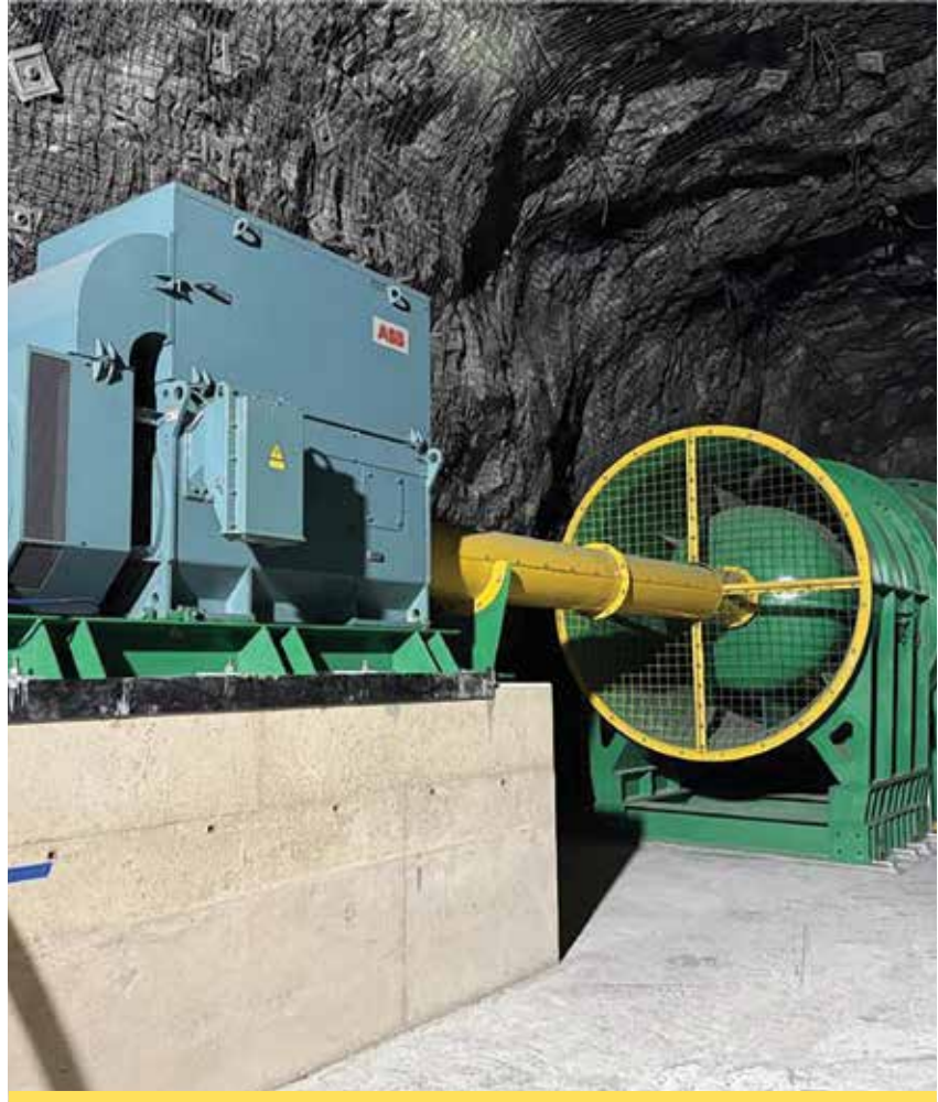
Beta Hunt Infrastructure Upgrade
