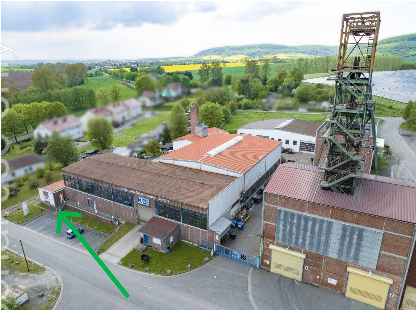
Location of South Harz's new office in Bernterode next to Shaft 1 in the Sollstedt licence area
