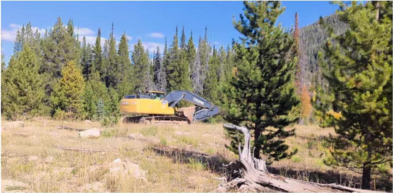
Figure 2 - Excavator on Thunder Mountain Road
